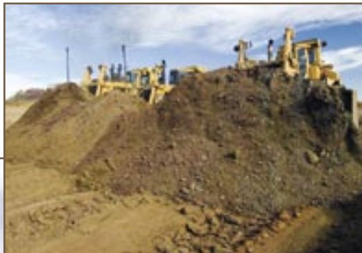
Garrett moved 170,000 cubic yards of dirt on the project.
