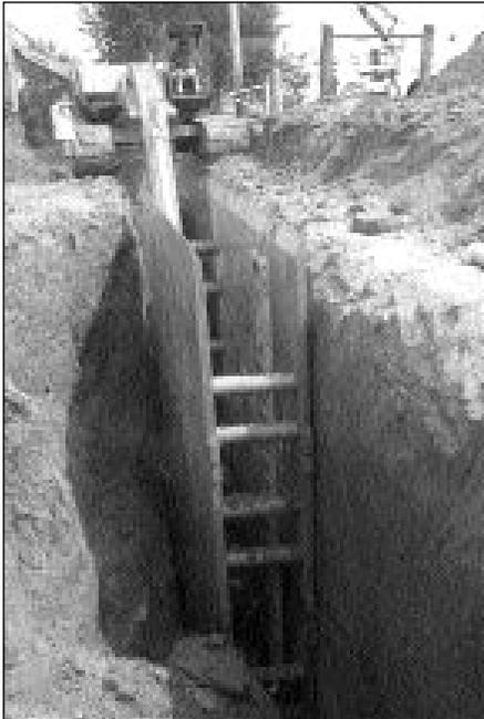
*A water and sewer contractor used three of TrenchSafety's 8'-high x 16'-long trench shields with 36" spreaders on a deep-sewer project near Hernando, Miss. The shields were stacked to a total of 24 feet of vertical protection. The cut was 27 feet deep.*
