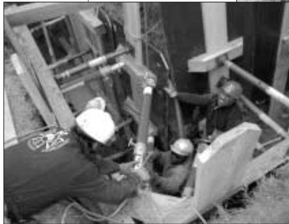
***hydraulic or air shores. The reason: the equipment is easily transported and adaptable to many different situations.***
