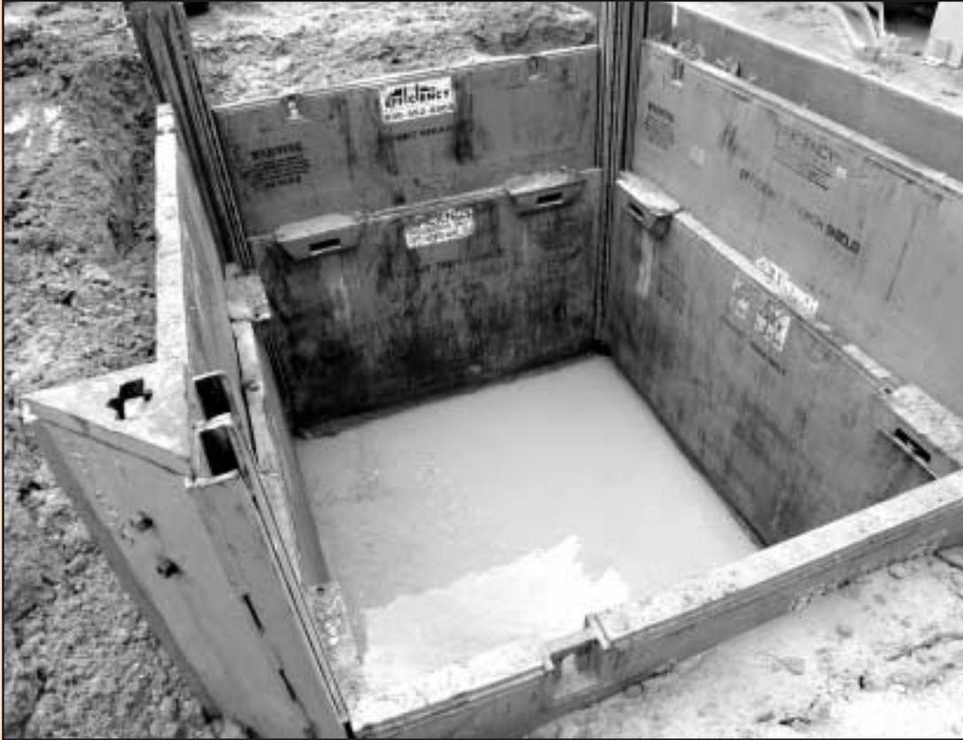
*In the left picture, the contractor was installing a tank at new power generating facility at the University of Mississippi, in Oxford. The system was 16' x 12' x 14' deep.*
