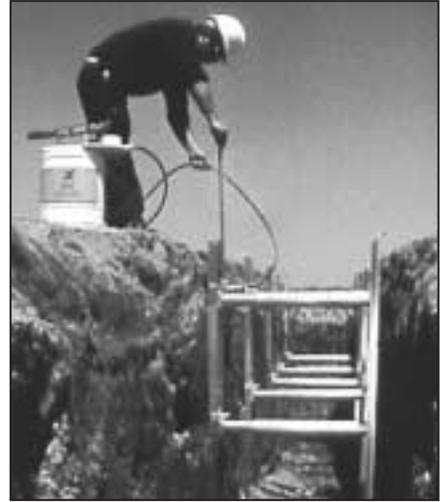
**3.** Shoring is now in place. Use release tool to disconnect hose fitting.
