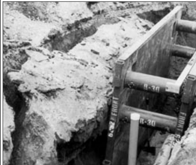
*At least two people's lives were saved by this trench shield when a massive chunk of soil gave way, slamming the side of this trench box.*
