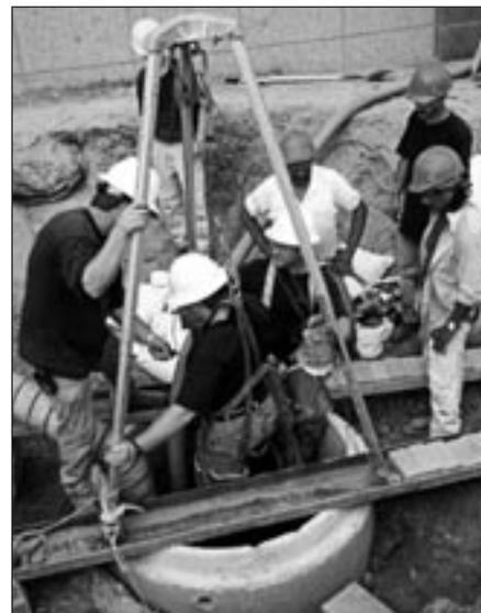
**Workers enter a very active 42" sanitary sewer at a recent project in Memphis. They had completed training, and conducted a thorough hazard analysis before entry. The workers utilized multiple ventilators, a gas monitor, a fall-protection/retrieval system, personal protective equipment, and a Confined Space Entry Permit to safely complete the job.**
