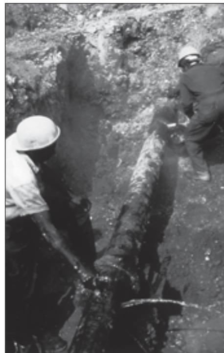
**Trenches may be classified as confined spaces or may contain hazardous atmospheres. It is important to be particularly cautious when operating gasoline- or diesel-powered equipment, or when working around swamps, leaking sewer lines, broken gas lines, near hazardous waste sites, and leaking petroleum tanks.**
