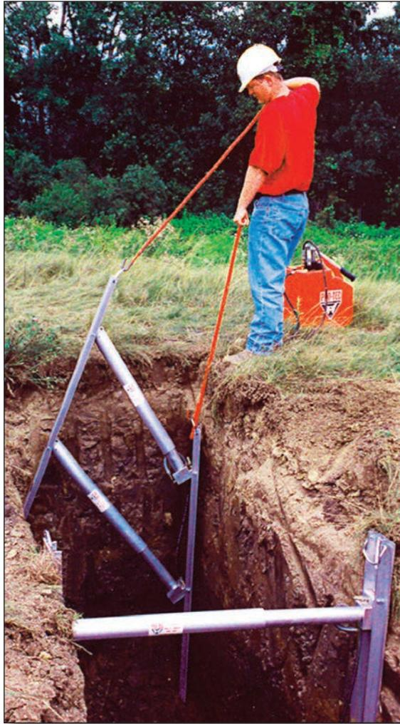
**Aluminum hydraulic shoring is an excellent choice for reducing costs and providing a safe workplace in many applications. The shores are light-weight and easily installed and removed by just one person.**
