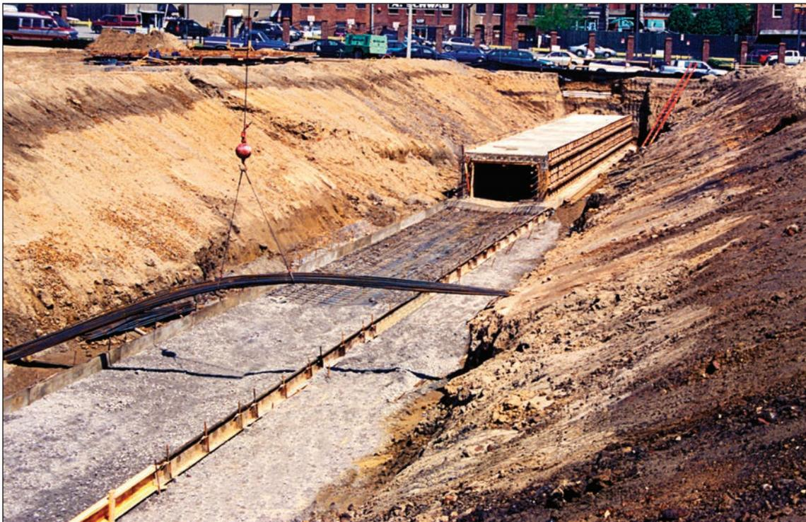
**Just imagine the time — and fuel — needed to excavate this large sloped trench. And, of course, all that soil is stored somewhere, and will have to be returned, the trench filled, and the surface restored.**
